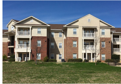
Clayton State University – Laker Village • Started Renovation – May 2021 • Completion Date – July 2022
