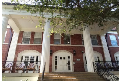
Georgia College & State University – Student Housing • Started Renovation – June 2021 • Completion Date – July 2022
